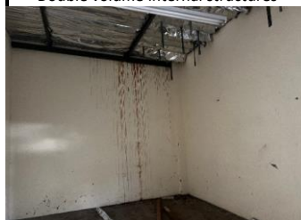
Sisalatation and roof leaks
